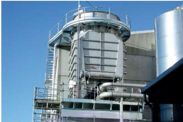
DAF is considered very efficient and is widely used in treating white water, TMP filtrates and wastewater for pulp and paper industry.
